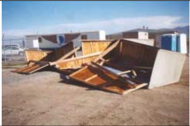
Wreckage of Tom West's hangar. Fortunately, Tom's Glassair was not inside.
