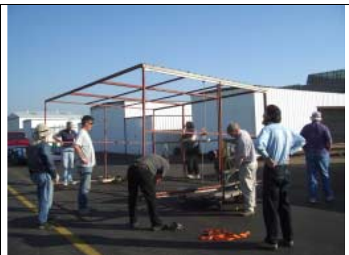
Preparing the hangar frame to go on the trailer at MYF.
